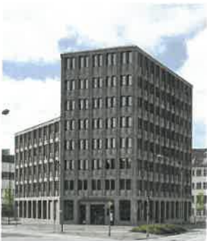
Taller element integrated into wider block (AOK Headquarters - Max Dudler Architects)
