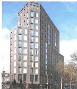
Sculptural massing form (H10 Hotel, Southwark - Maccreeanor Lavington Architects)
