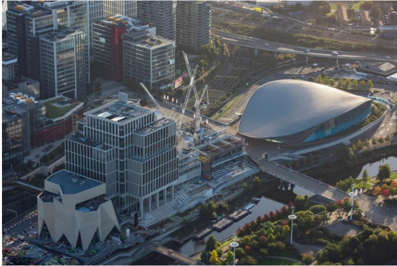
Aerial shot of East Bank © Queen Elizabeth Olympic Park
