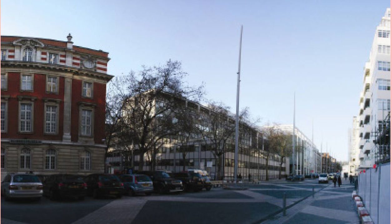
Site as existing (Image: Jerry Tate Architects)
