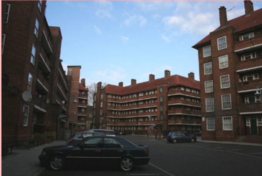
Site as existing (Image: Jerry Tate Architects)
