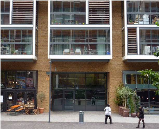
Residential entrance located adjacent to retail units – Dalston Square
