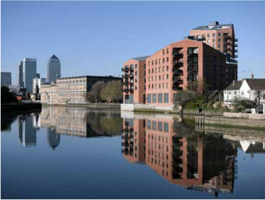
Working with the geometry of the site and its constraints has influenced a contextually driven form and a responsive massing. Lock Keepers, Bromley-by-Bow, Gillender Street, Allies and Morrison, Photography: Nick Guttridge
