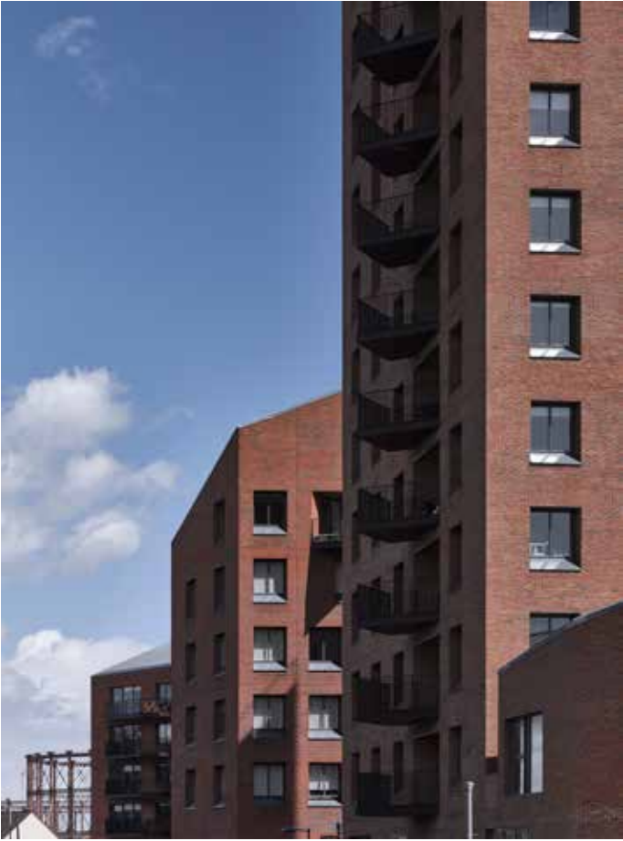
A 1 bed arrangement that minimises corridor but allows for a generous hall with direct views and daylight as you enter. Lock Keepers, Bromley-by-Bow, Gillender Street, Allies and Morrison, Photography: Nick Guttridge
