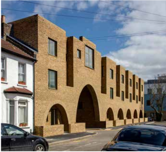
Homes can be a backdrop for everyday life, creating great streets and strengthening the inherent identity of a place. Worland Gardens, Peter Barber Architects, Photography: Morley von Sternberg FRIBA
