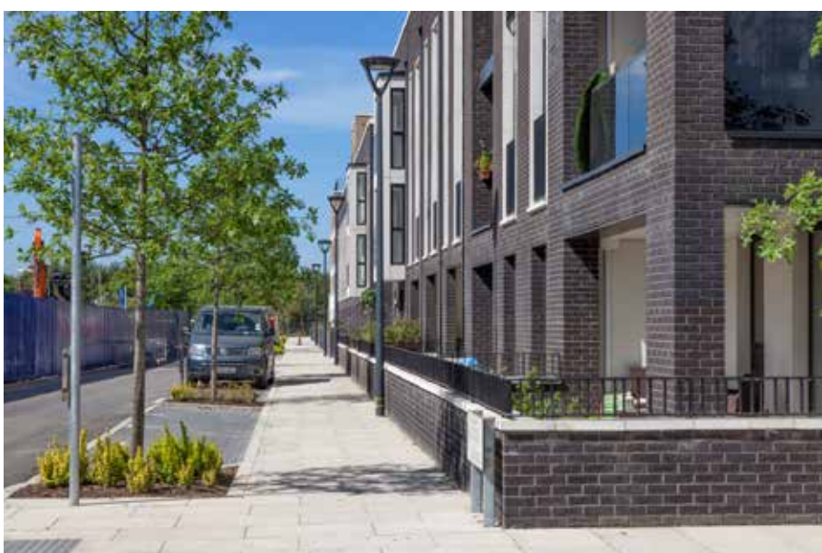
Left: Well-integrated car parking can activate streets, while careful material treatment and planting can reduce perceived road widths and help to mitigate the visual impact of cars. Villiers Gardens, Chobham Manor, PRP and muf architecture/art, Photography: PRP Right: Streets should be inclusive places of cultural exchange and expression of the wider community. Narrow Way Pedestrianisation, Studio Weave Architects, Photography: Studio Weave Architects
