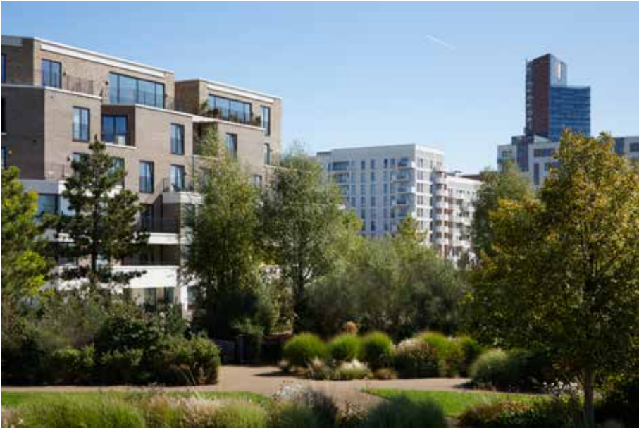
The homes on Olympic Park Avenue reference the civic qualities of a Nash terrace, creating a strong built form as a backdrop to the wild planting of the North Park. Park View Mansions, Chobham Manor, Haworth Tompkins and muf architecture/art, Photography: Jack Hobhouse
