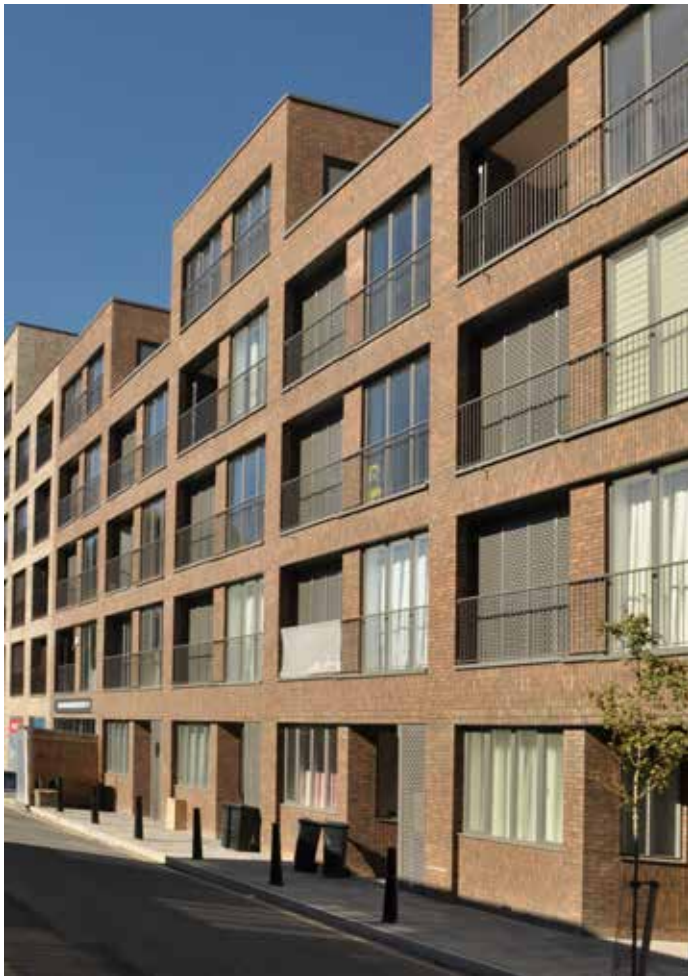
Left: Simple building forms with strong roofscapes can give the street rhythm, structure and hierarchy. 85 Monier Road, Hawkins\Brown, Photography: LLDC
