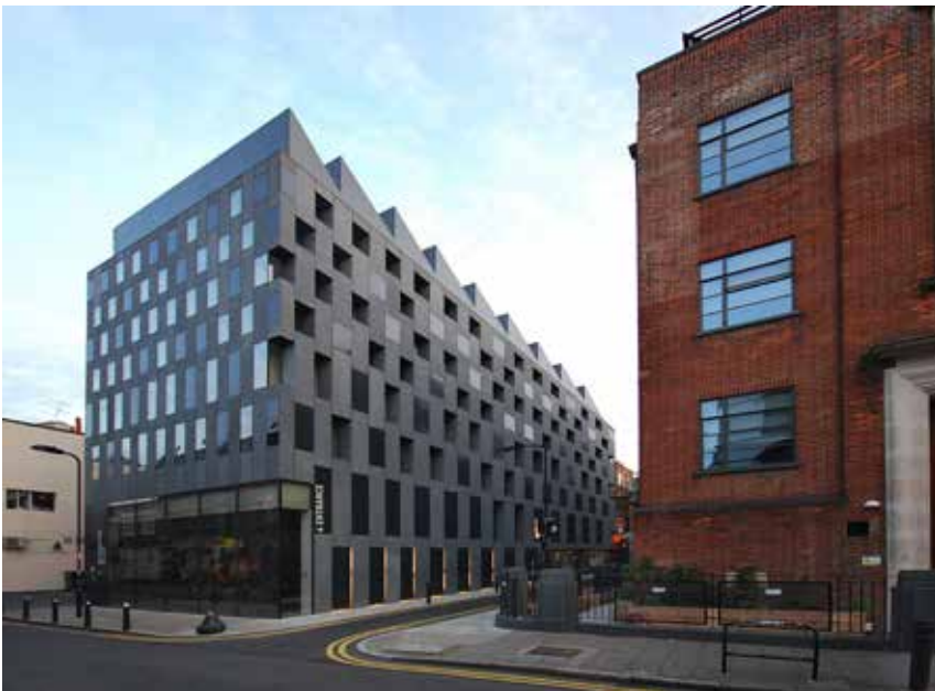
Strong massing can be used to make bold and highly legible urban forms, with a subtle variation in articulation providing greater expression. Rivington Place, Adjaye Associates, Photography: Lyndon Douglas
