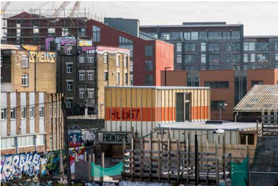
Care and attention should be given to all buildings; this community centre uses form, materials and textures to give a playful and meaningful expression to temporary use. Hub 67, LYN Atelier, Photography: LLDC
