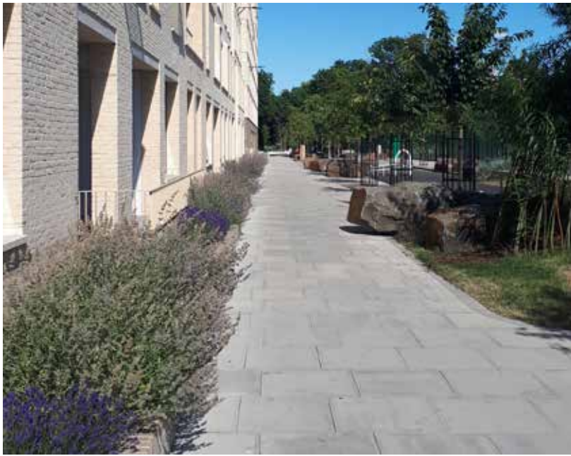
Planting should be used at important thresholds to create hierarchy, and soften the transition between public and private spaces. Kings Crescent Estate Phases 1 & 2, muf architecture/art, Karakusevic Carson Architects and Henley Halebrown, Photography: LLDC
