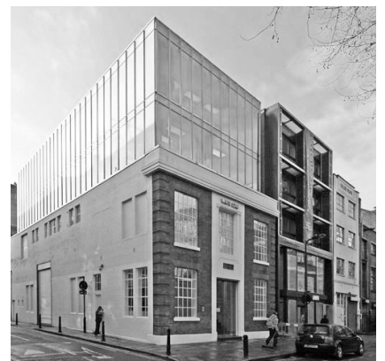
White Cube, Hoxton, MRJ Rundell + Associates: A robust structure retained and renewed
