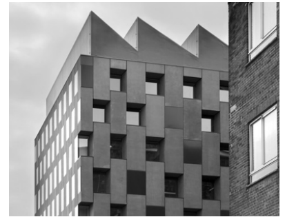
Iniva, Rivington Place, London, Adjaye Associates: The deep reveals add drama to the asymmetrical grid of window openings which pattern the facade as a whole
