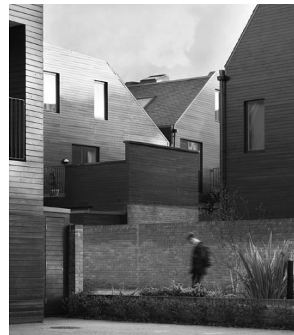
Newhall Be, Essex, Alison Brooks Architects: Design is inspired by the local vernacular but uses crisp, contemporary detailing.
