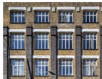
Clarnico Works: Windows align vertically within engineering brick piers
