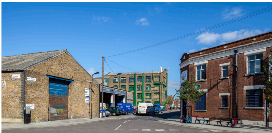
Above: Wallis Road Corner
