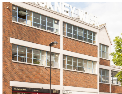
Oslo House: An articulated structure frames brick infill panels and strip windows
