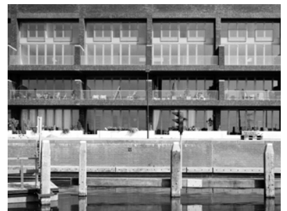
Ijburg Blok 4, Amsterdam, Macreanor Lavington: Windows align vertically within a brick facade
