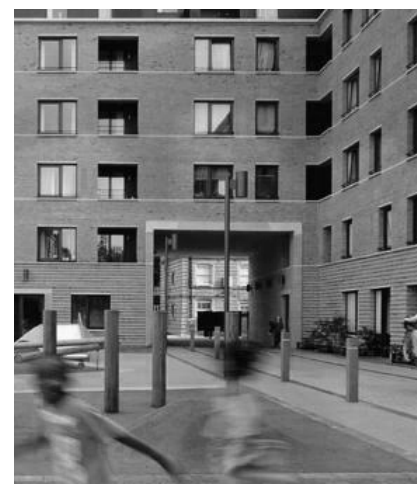
Peabody Avenue, Pimlico, London, Haworth Tompkins: The internal yard is connected to the street by a double height opening through the building
