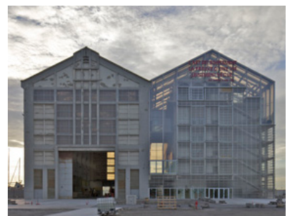
FRAC Nord-Pas de Calais, Dunkirk, Lacaton + Vassal: Robust vertical scale and repetition
