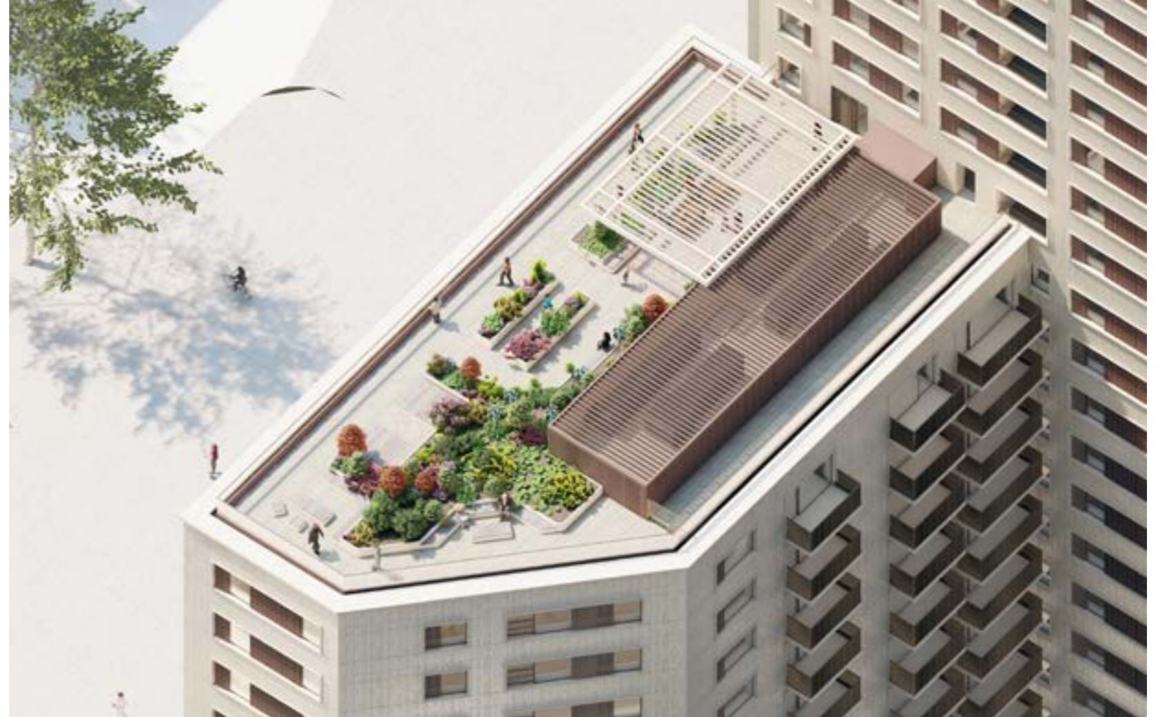
Fig.95 Aerial View from N19 Roof Terrace
