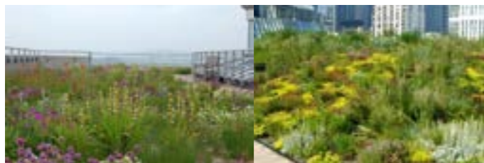
Semi-intensive green roof with a somewhat deeper substrate, creating the opportunity for growth of some shrubs (but bringing with it a greater maintenance requirement)
