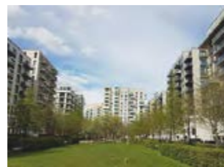
Fig.2 Typical East Village perimeter blocks on Mirabelle Gardens
