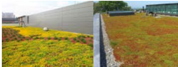
Extensive green roof with less than 200 mm of soil or substrate.
