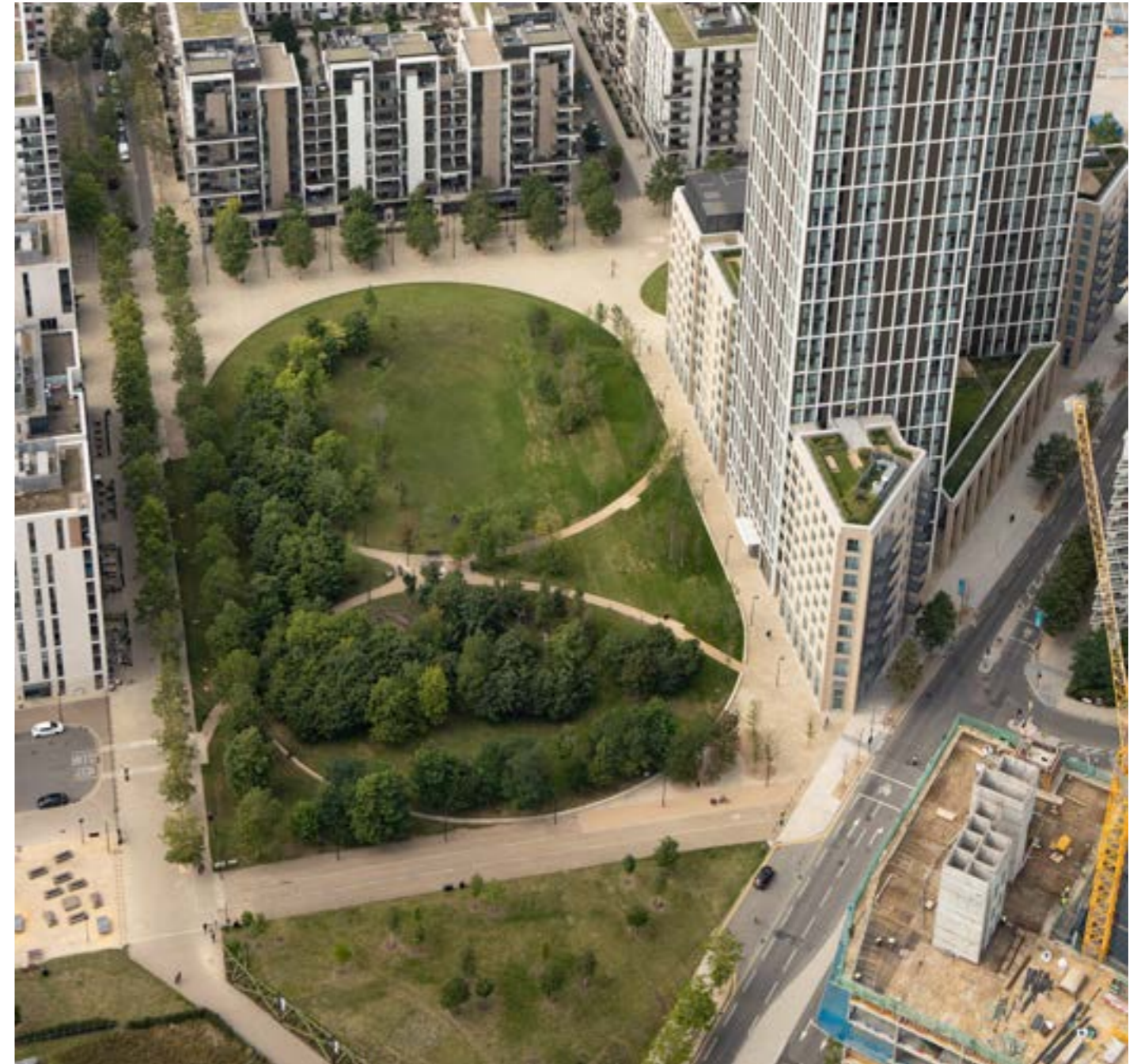
Fig.196 Aerial view of the site showing adjacent existing Victory Park
